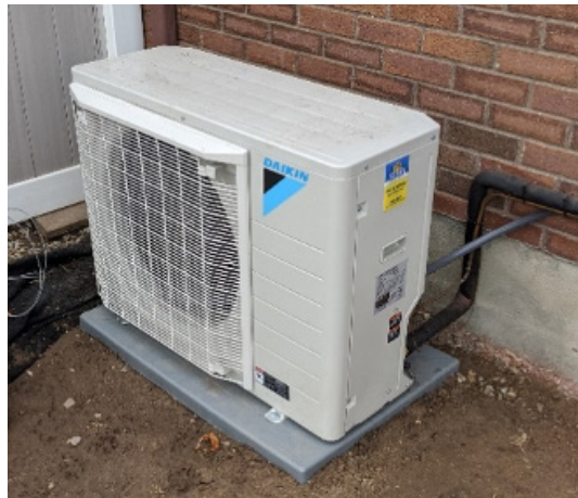
Quality Inspection of New Dual Fuel Heat Pumps
